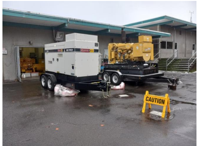
The hatchery has a main generator inside the building that is currently running. The generators here are back-ups.
