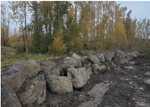
Large rock barrier prevents illegal vehicle access to Wilsonville Fishing Pond
