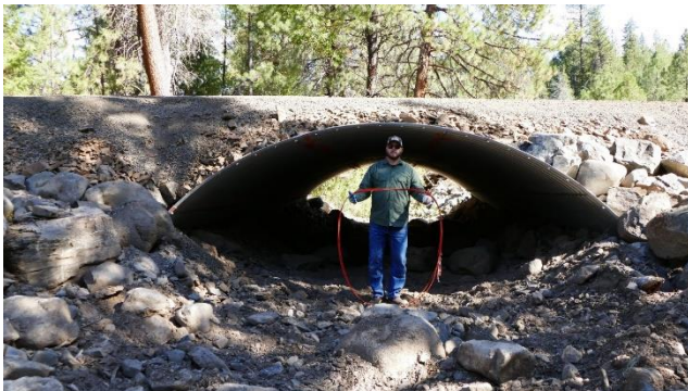
The orange rope represents the size of the previous culvert that was replaced
