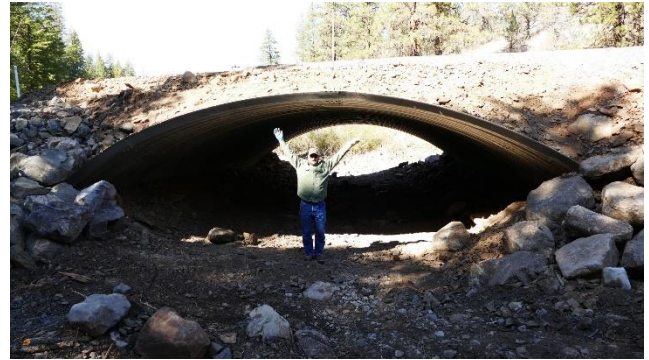
New thirty-three-foot wide, open bottom culvert that replaced two, six-foot wide culverts
